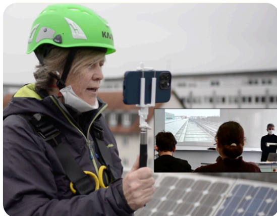
Christina from SOFS, livestreaming to a class while doing an annual inspection of the solar panels
